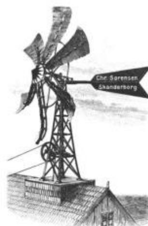
Figur 10: Right: The conical wind catcher rotor as a roof mill with only six sails.
