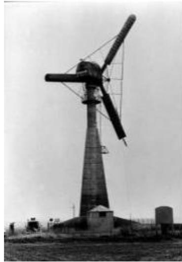
Figur 26: Right: Photograph of the Gedser turbine. The first 3-wing AC mill with tip safety brakes.
