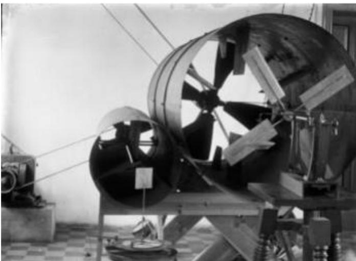
Figur 14: Left: Photograph of the wind tunnels. One with diameter 1 m and one with diameter 0.50 m.
