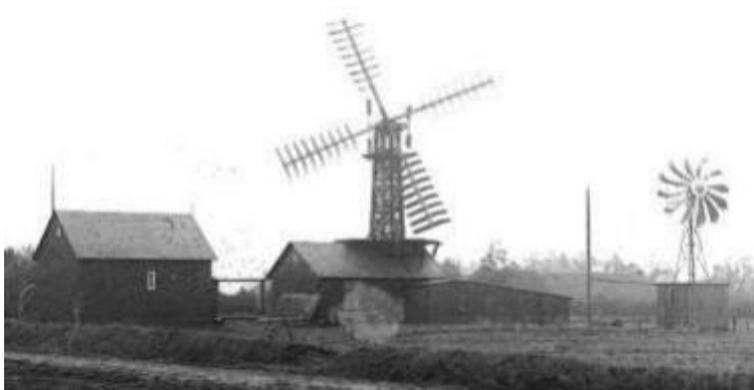
Figur 9: Left: This photograph from 1896 shows the "conic wind cather" with twelve sails.
